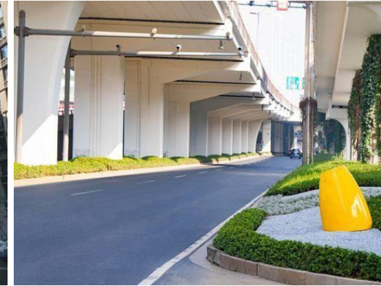
Elevated bridge obstructions
